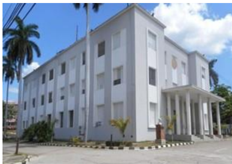
Figure 1: View of the first central building.
